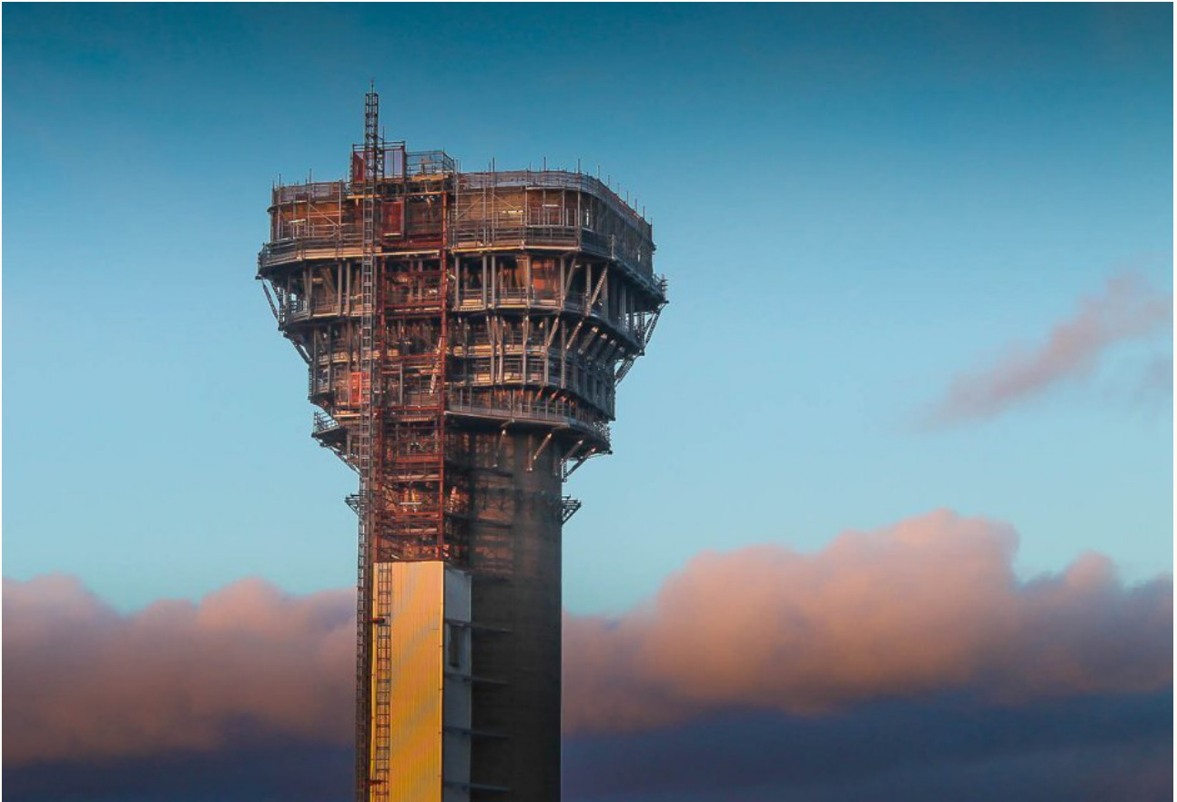
The diffuser on the Windscale Pile 1 chimney during decommissioning. The filter in this distinctive structure reduced the radionuclides released in the 1957 fire.
