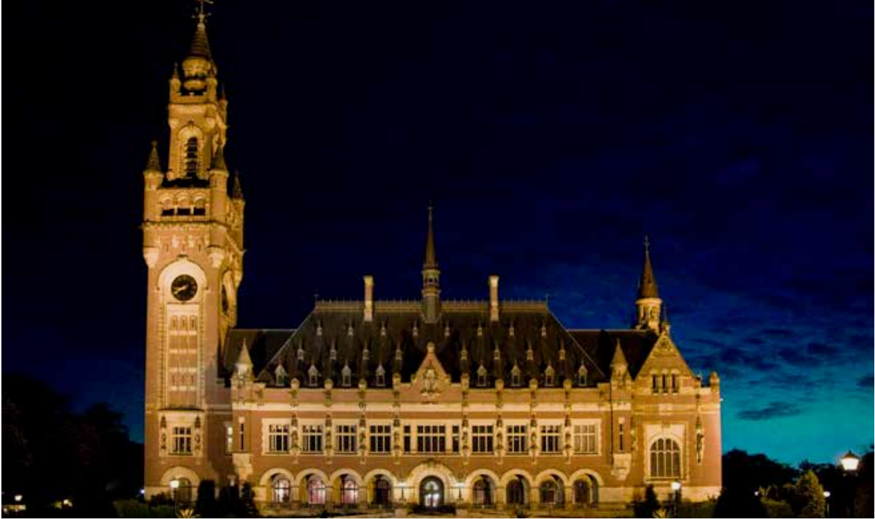
The Peace Palace in the Hague, the Netherlands, housing the International Court of Justice.
